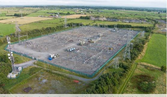
Example of air insulated switchgear (AIS) substation - Cashla 220 kV Substation
