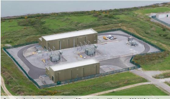
Example of gas insulated switchgear (GIS) substation - Kilpaddoge 220 kV Substation
