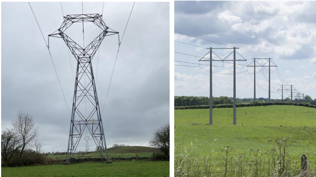
Figure 2.3: Lattice Tower (left) and a Photomontage showing Composite Poles (right)
