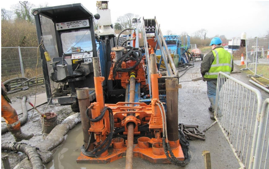
Figure 32 - HDD Rig - East West Interconnector
