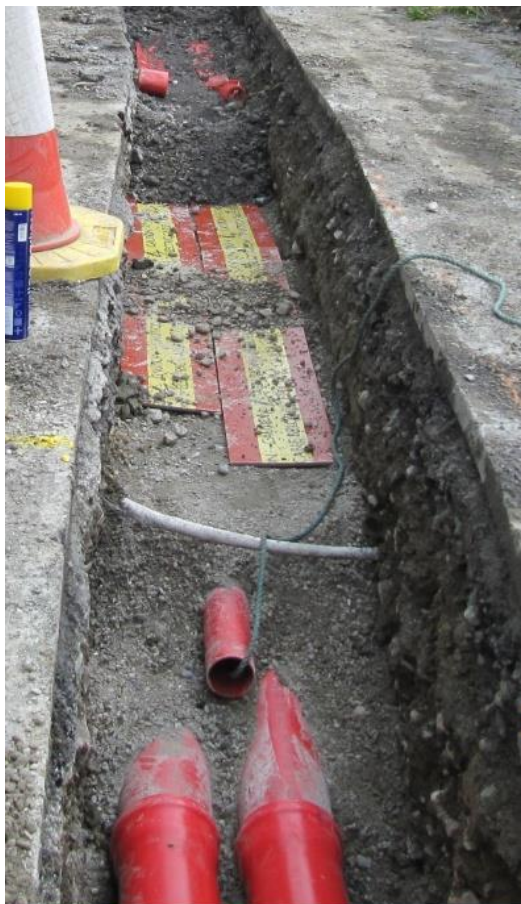
Figure 29 - Cable Trench – East-West Interconnector
