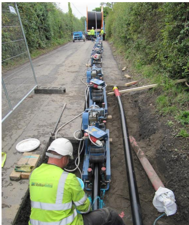
Figure 30 - Cables Being Pulled Into Conduit
