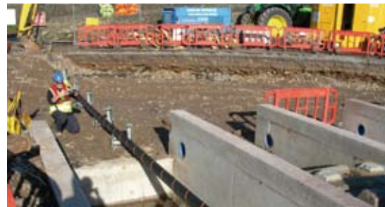
Aghada - Raffeen cable construction coming onshore
