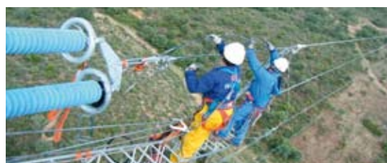
Crew restringing HTLS Conductor
