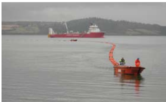
Cable laying in Cork Harbour
