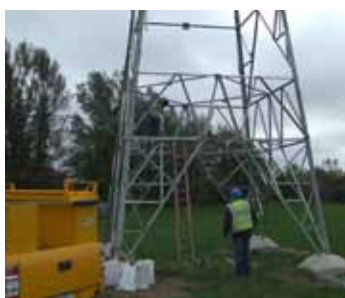
Tower construction on the Gorman - Meath Hill 110kV Line
