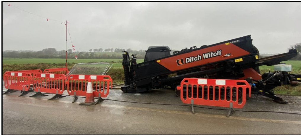
Figure 2-11 - HDD rig drilling a pilot hole for HV UGCs
