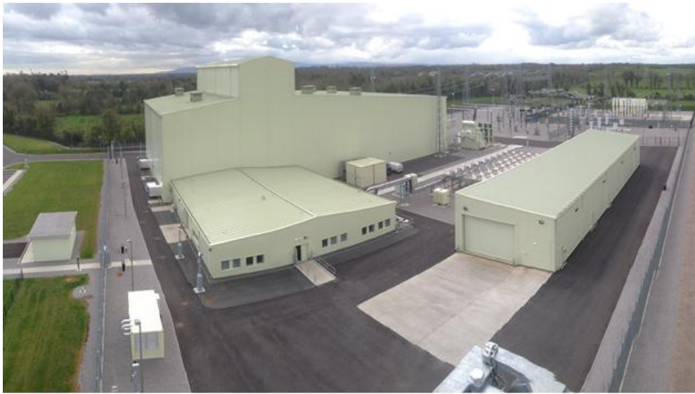
Figure 4-1 Existing VSC Converter Station for the East West Interconnector at Woodland, County Meath
