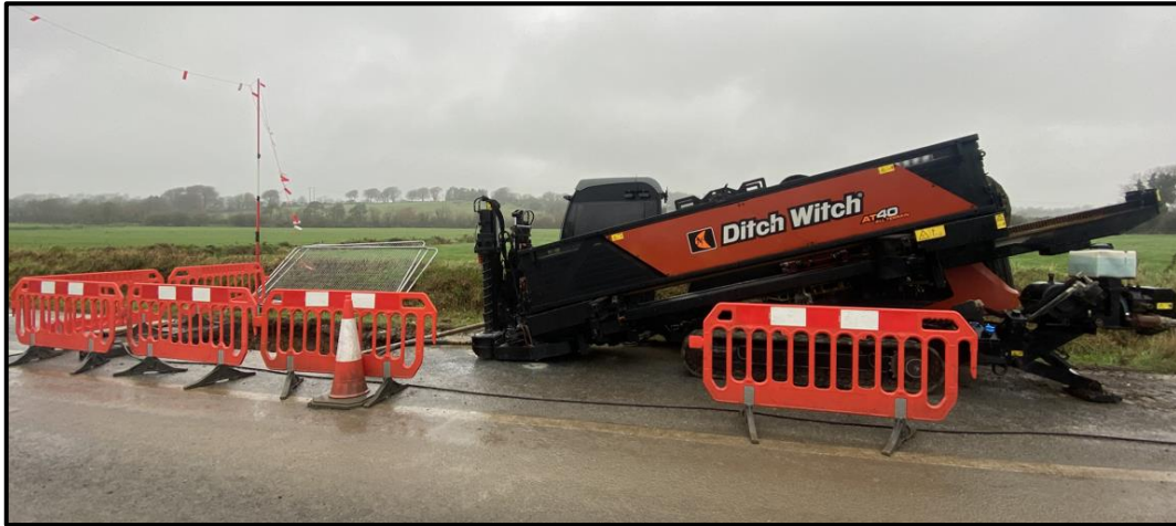
Figure 2-8 - HDD rig drilling a pilot hole for HV UGCs
