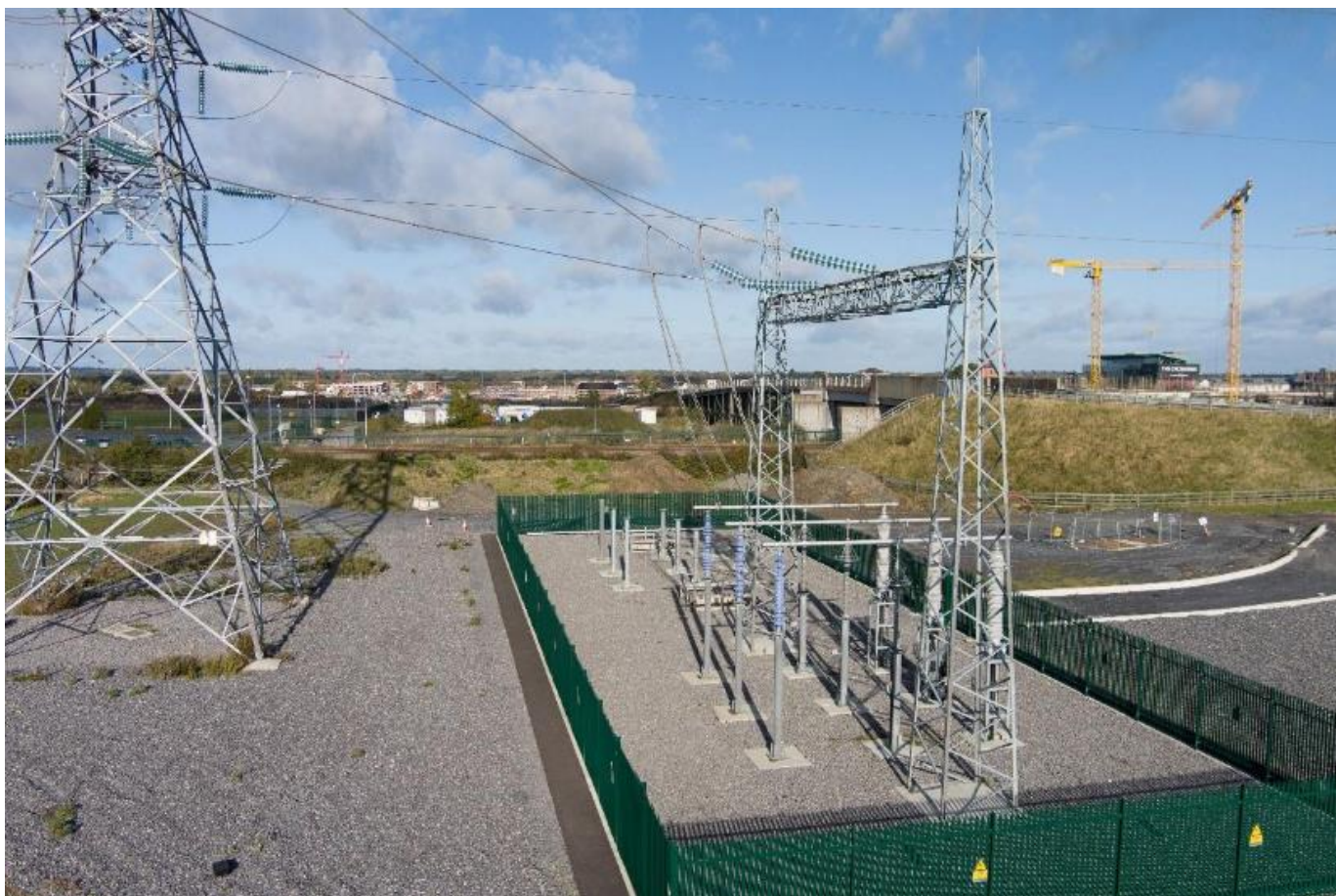
Figure 2-9 - 220 kV OHL to UGC Interface Compound
