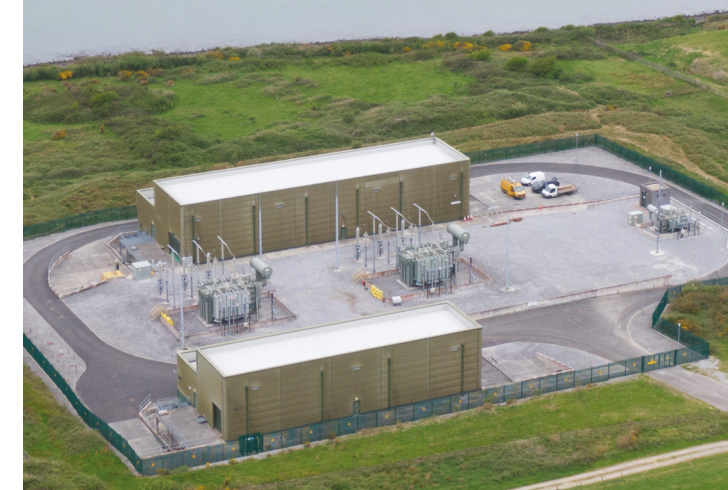
Technology option 1 - Gas Insulated Switchgear (GIS) Substation
