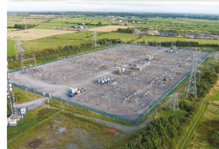
Technology option 2 - Air Insulated Switchgear (AIS) Substation
