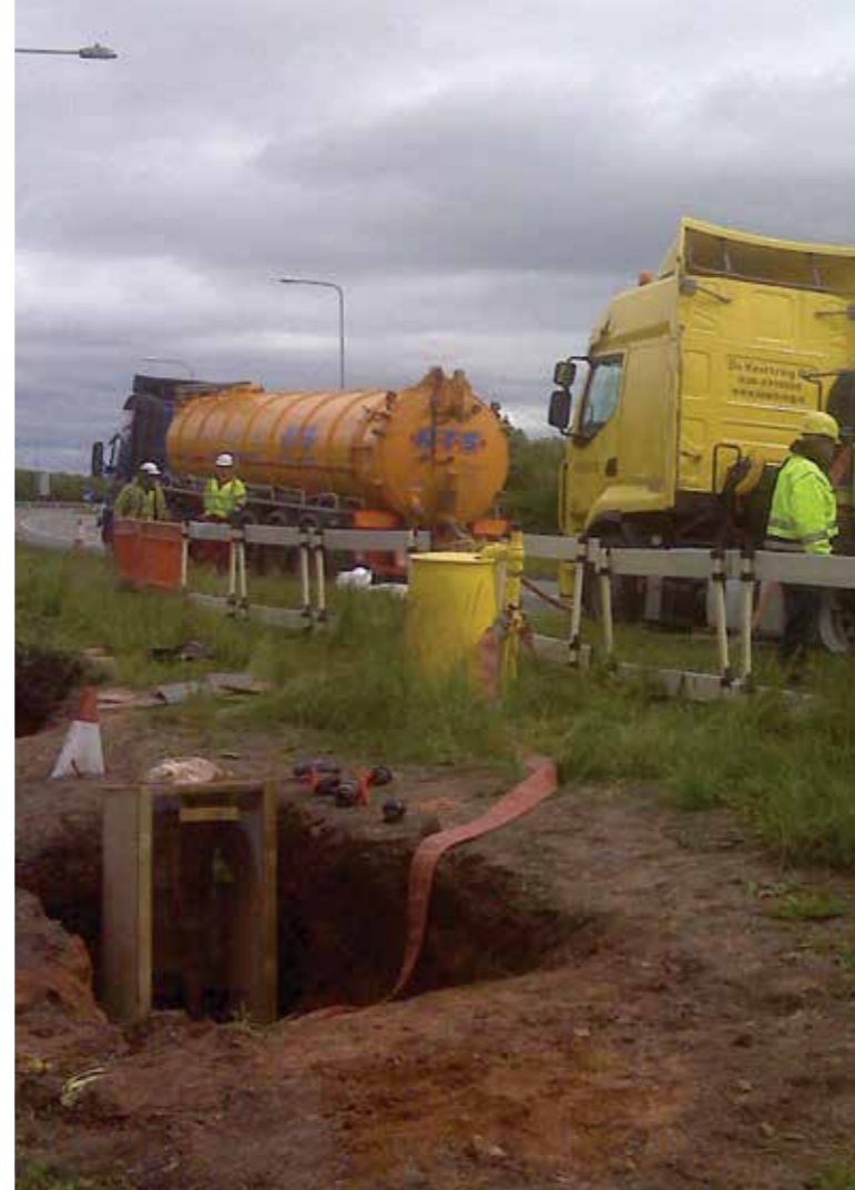
FIGURE 5: INSTALLATION OF CLAY GROUT IN THE DUCTS
