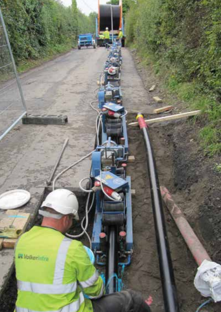
FIGURE 4: INSTALLATION OF CABLE INTO THE DUCTS
