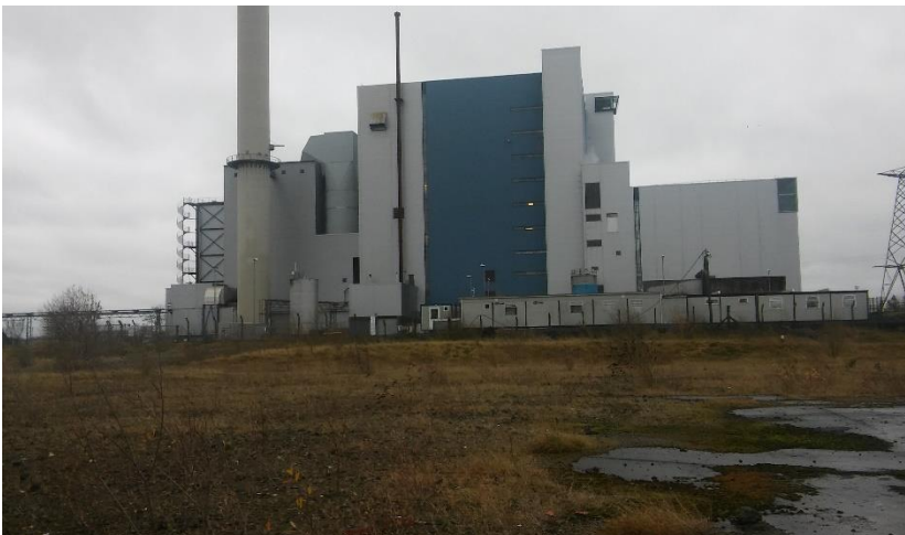
Figure 17: Lough Ree Power Station
