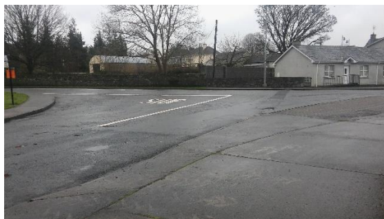
Figure 14: Exiting on to the N63 from the Proposed Development site
