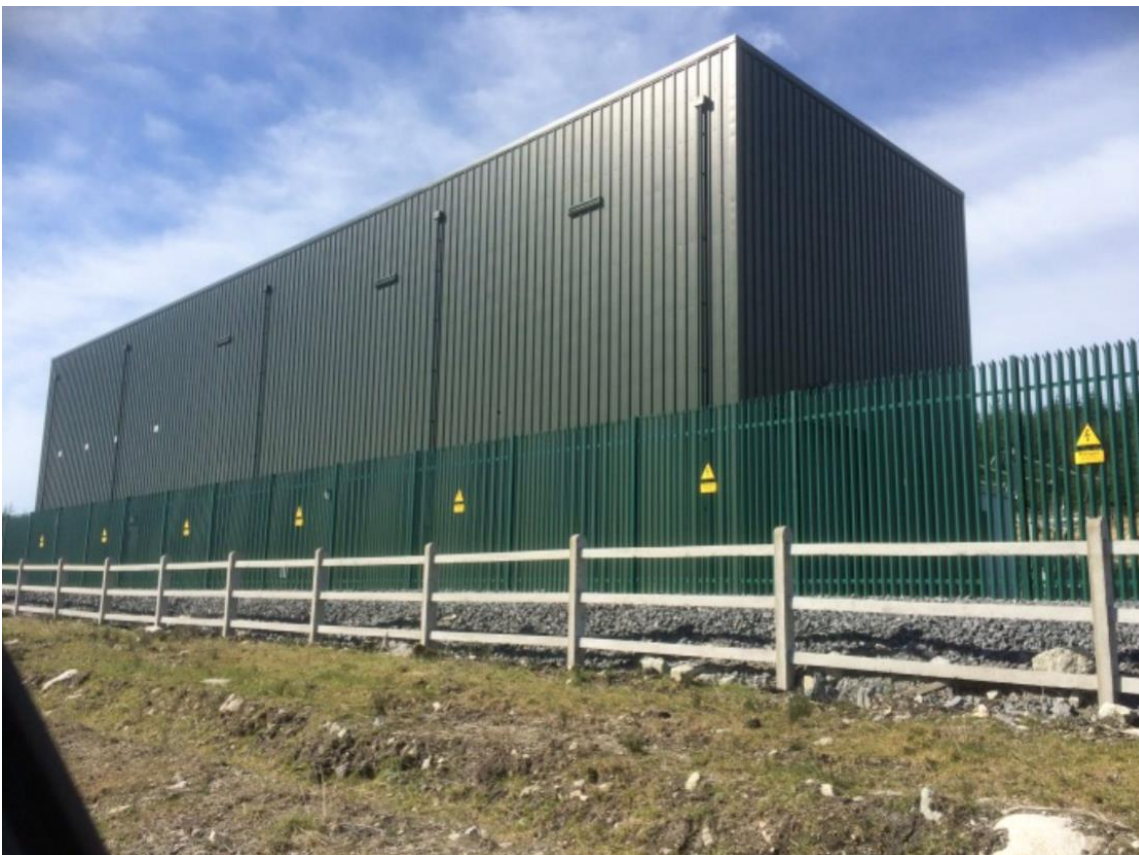
Figure 25: Typical 110 kV GIS Substation building
