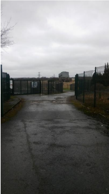
Figure 11: Lanesboro 110 kV Substation Entrance and Boundary Fencing
