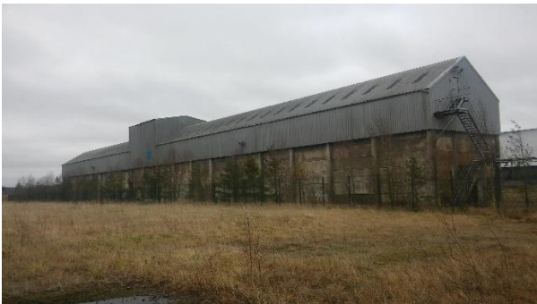
Figure 20: NIAH Structure (Reg. No. 13310017)
