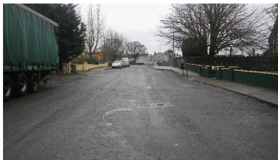
Figure 10: Access Road (South Orientation)
