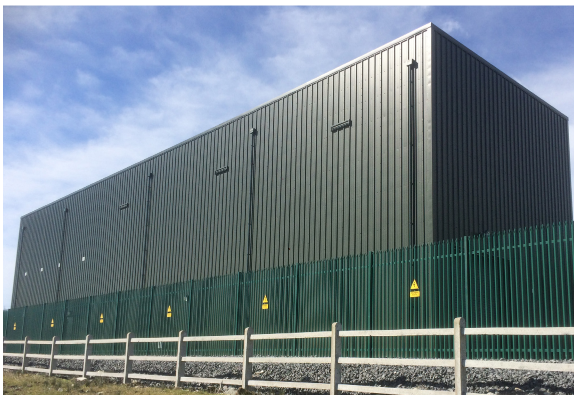
Typical GIS substation building
