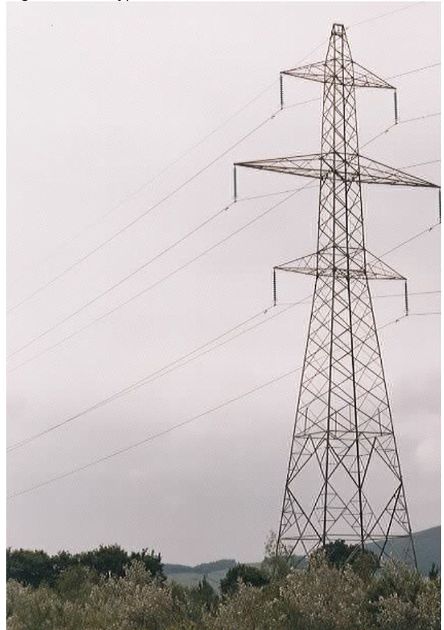
Figure 1.10: Typical 110 kV DC Tower
