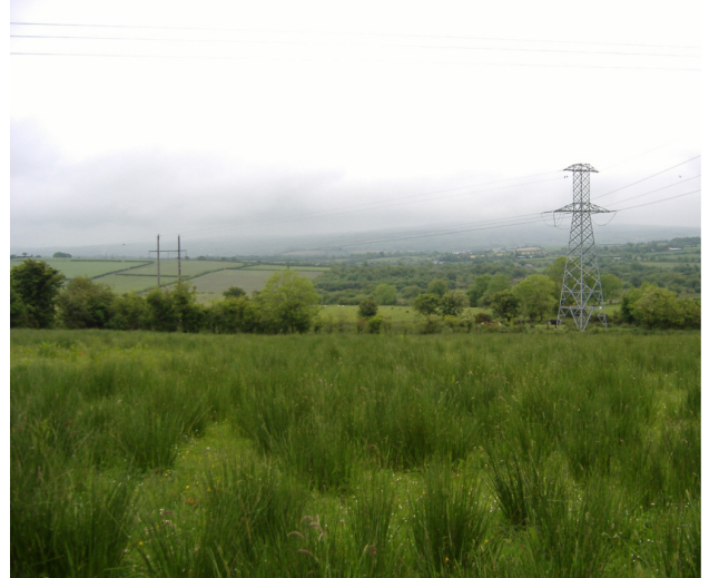
Figure 1.8: Typical 110 kV Steel Angle Tower
