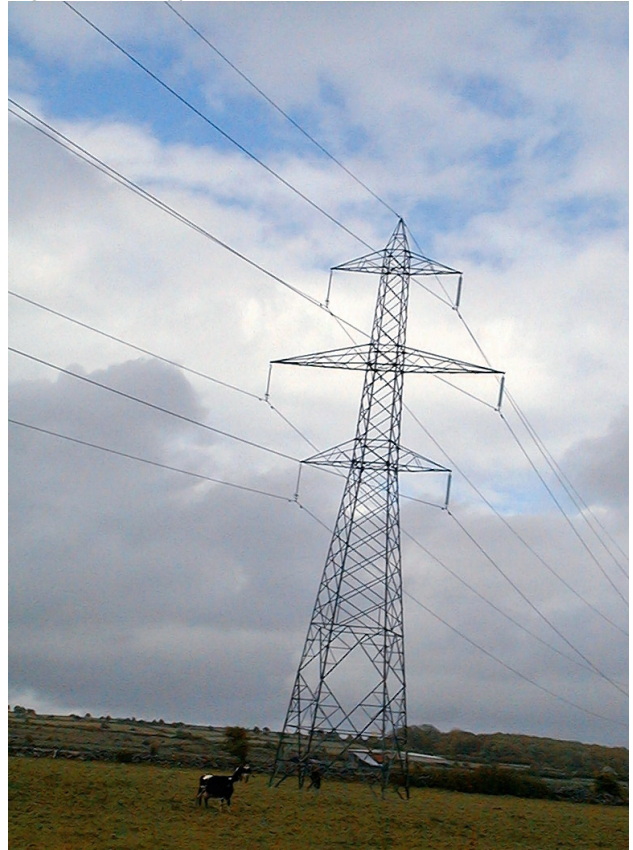
Figure 1.14: Typical 220 kV DC Tower
