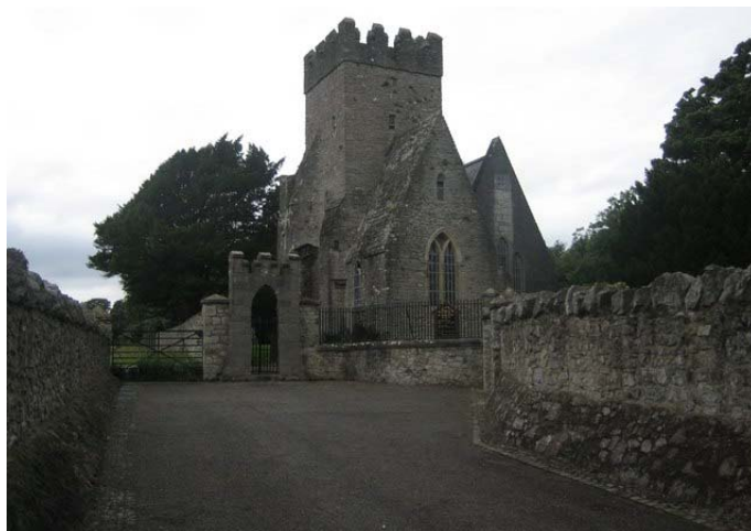
Figure 8: St Doolagh's Church (within Study Area)
