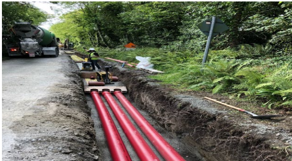
Figure 6: A typical cable duct installation in the road
