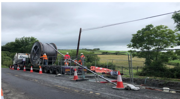
Figure 8: Cables being pulled into the ducts and jointing bay
