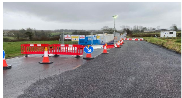
Figure 9: A typical passing bay in operation during cable jointing
