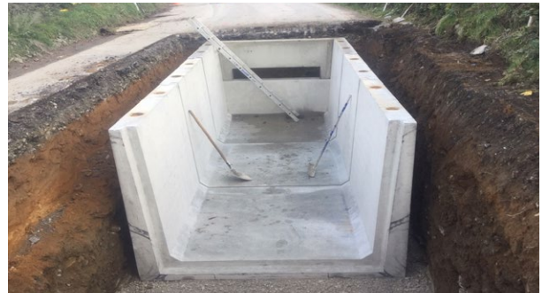
Figure 7: A typical jointing bay where cables are connected
