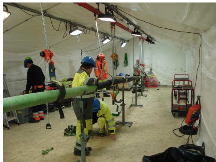
Figure 2 - Repair work on HVDC cable: Moyle Interconnector
