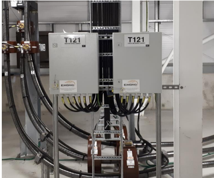
Photo 1 Ring CTs and Metering marshalling kiosk
