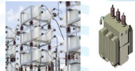
Capacitor Banks provide reactive power and can increase voltage
