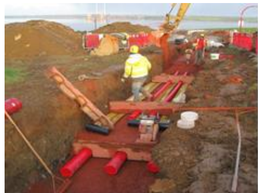
Figure 2-8: Typical Trench for HVAC Underground Cable
