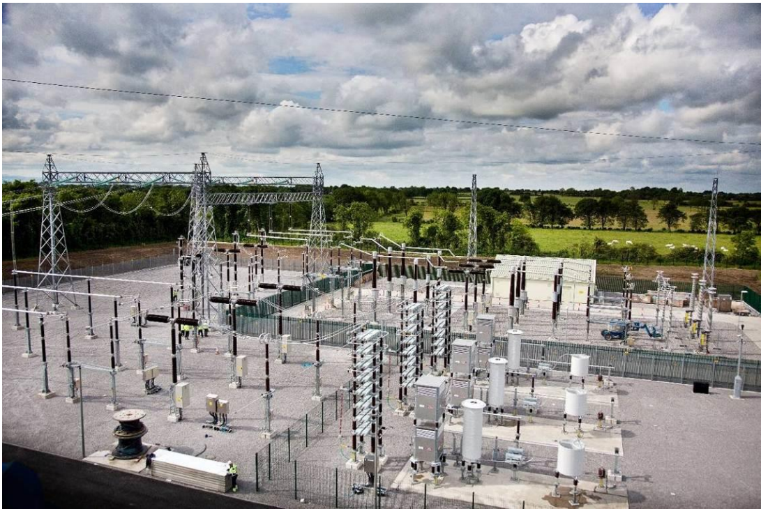
Figure 2-6: Outdoor HV Equipment at HVDC Converter Station (source: ABB)
