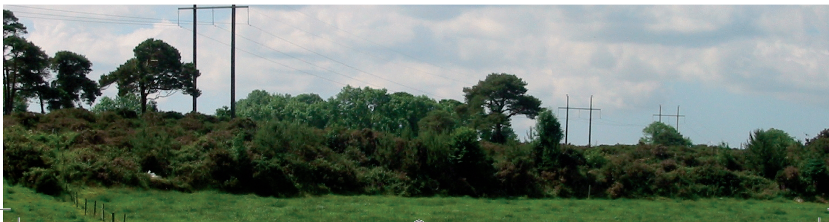
Picture of existing Dunmanway-Macroom 110kV line.
