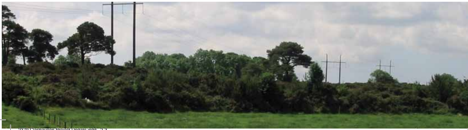
Fig.1 Existing Dunmanway-Macroom 110kV line
