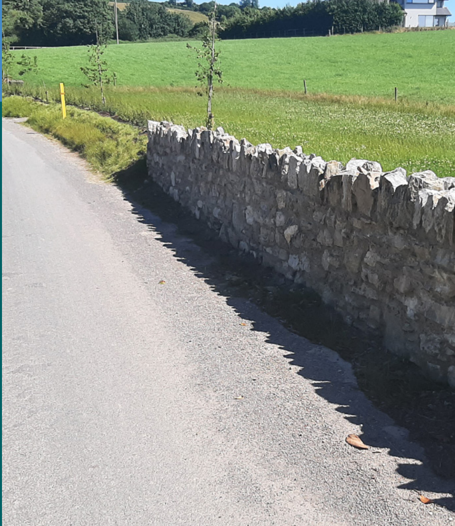
Image: Typical road reinstatement following installation works
