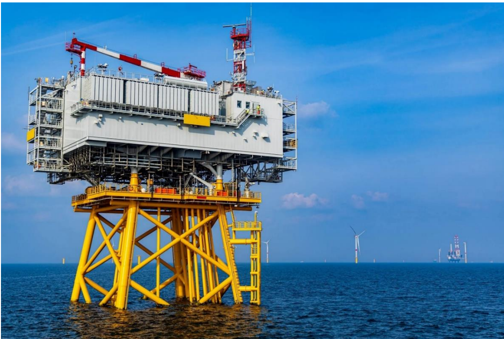
Figure 2.1: Typical Enclosed-type OSS Platform
