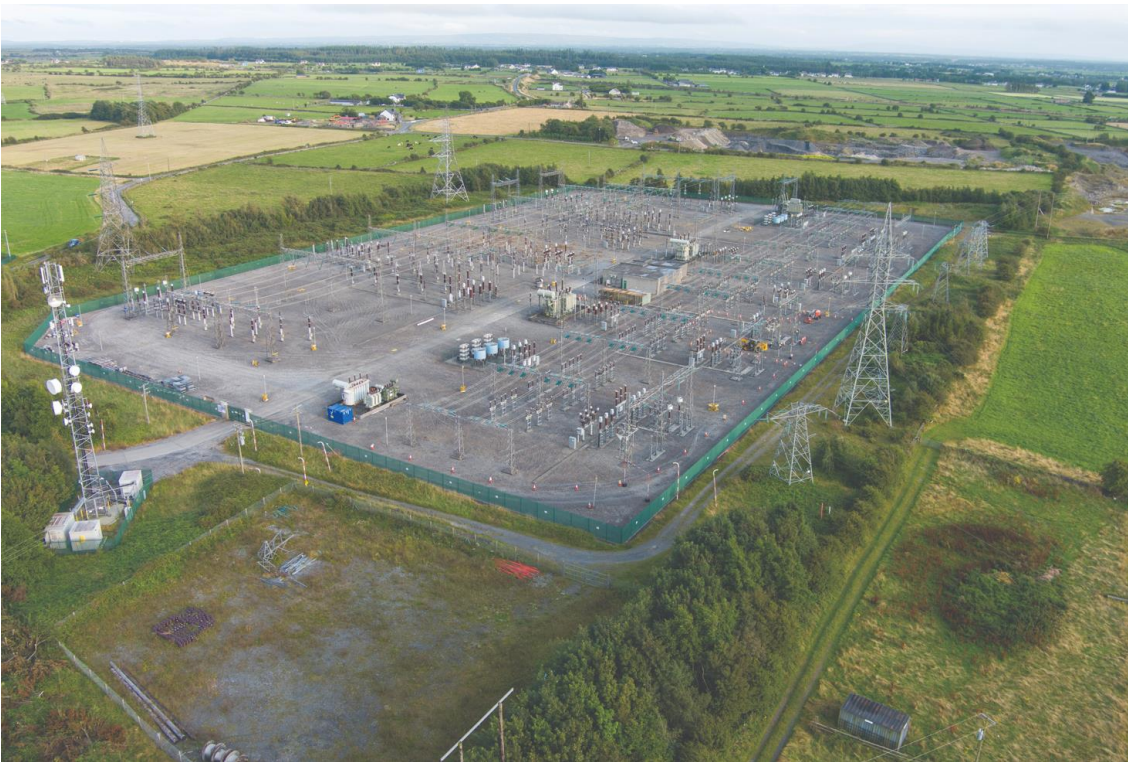
Figure 2.3: Typical AIS Substation
