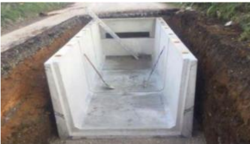
Figure 2.5: Typical Joint Bay
