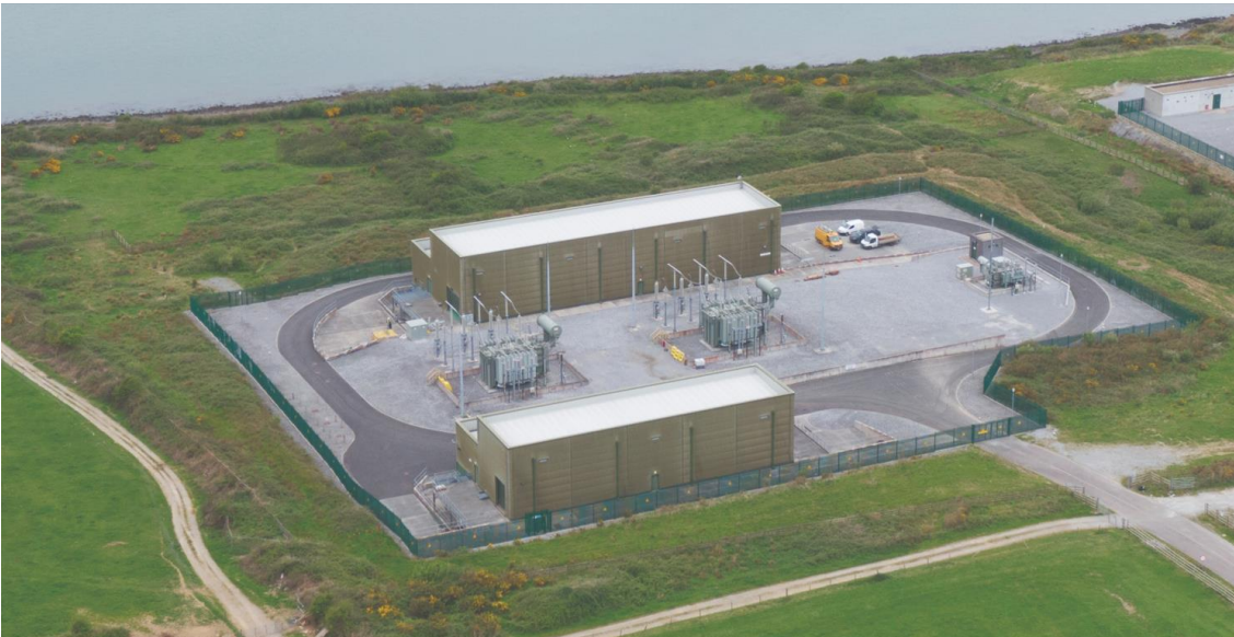
Figure 2.4: Typical GIS Substation
