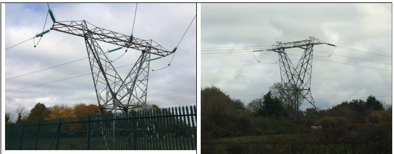
Figure 3.18 : Single Circuit 220kV Section / Angle Towers (Dunstown-Woodland)
