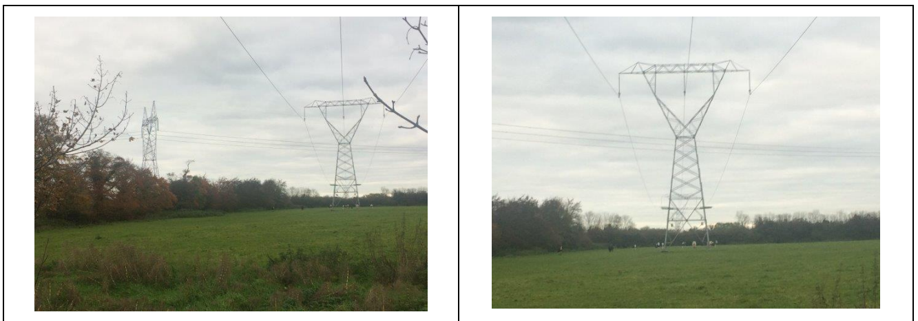
Figure 3.4 : Existing Maynooth - Gorman 220kV circuit passing beneath Old Street – Woodland 400kV circuit
