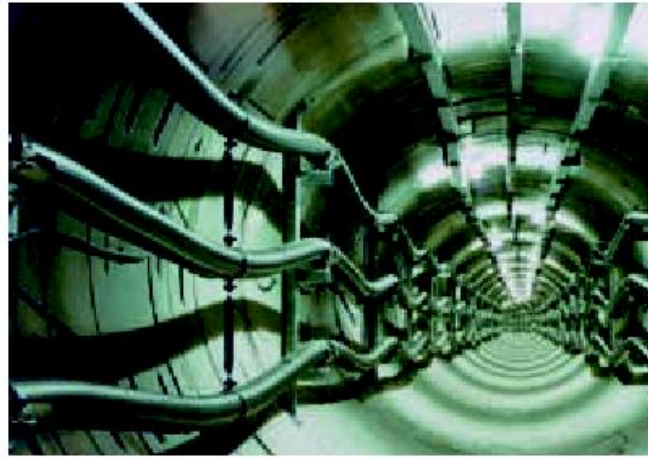
Tunnel (normally in urban areas)
