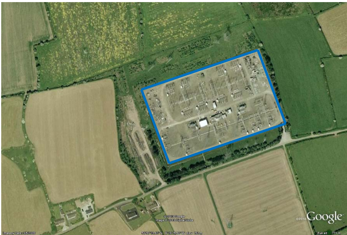
Figure 7.8: Knockraha Substation Site (Aerial View)
