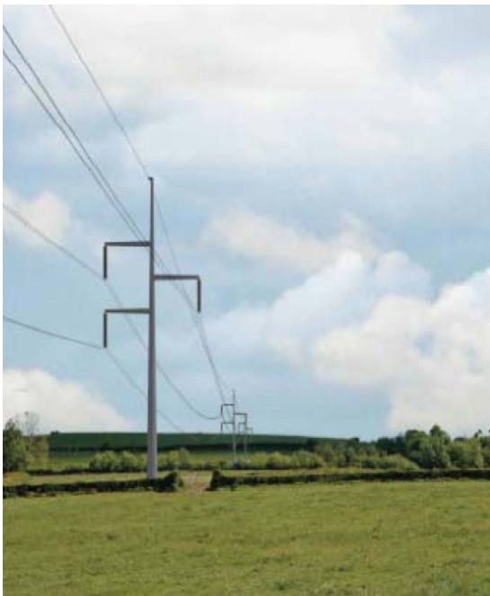
Single circuit 400kV Monopole
