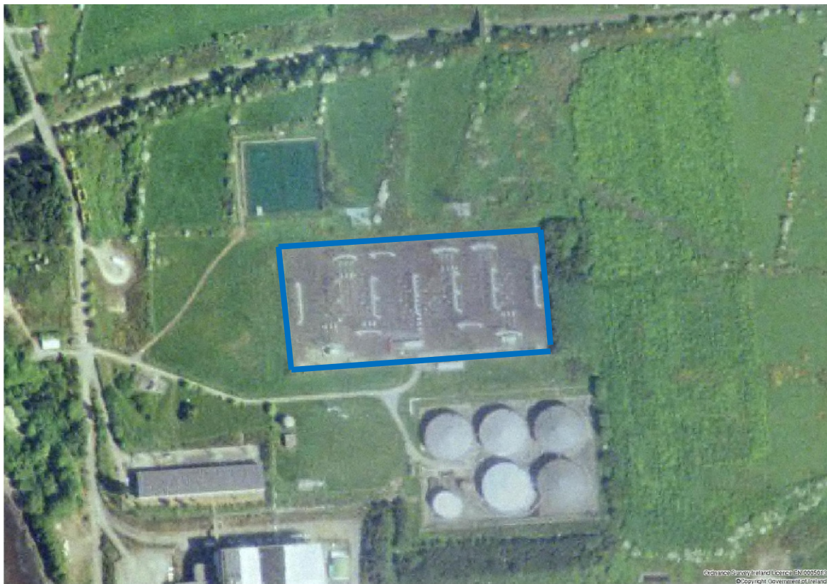
Figure 7.5: Great Island Substation Site (Aerial View)
