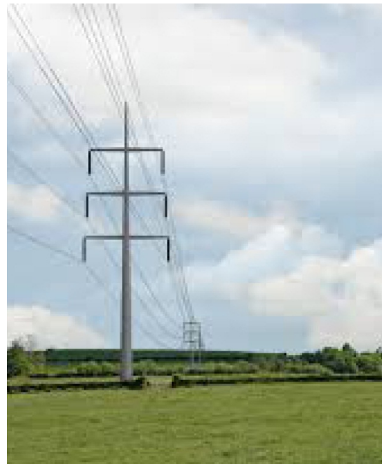
Double circuit 400kV Monopole
