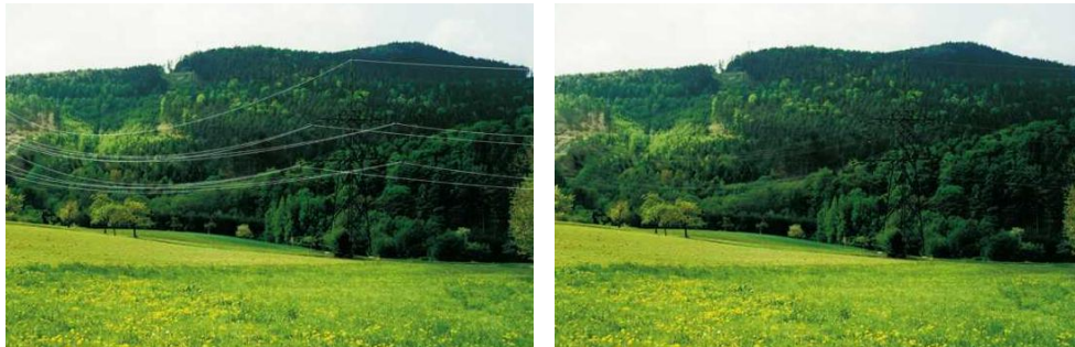
Figure 12: Application of coloured conductors left before, right after application
