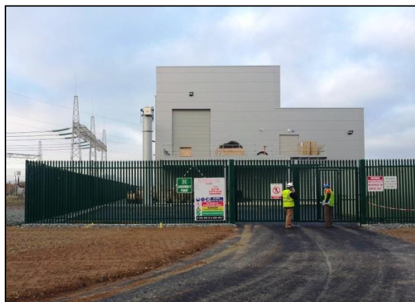
Plate 3-2 Typical Indoor GIS Substation
