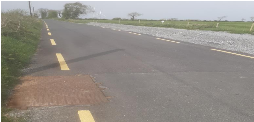
Figure 4.2: Re-instated Road following joint bay installation
