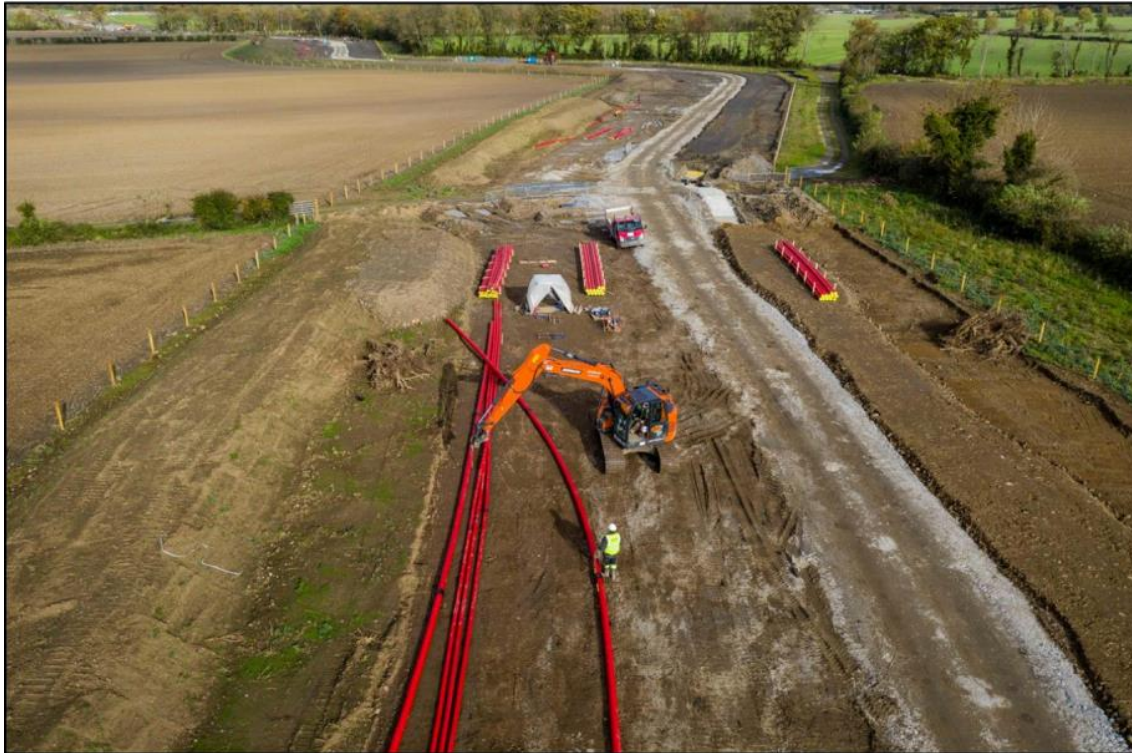
Figure 4.4: Typical UGC Construction in Agricultural Lands
