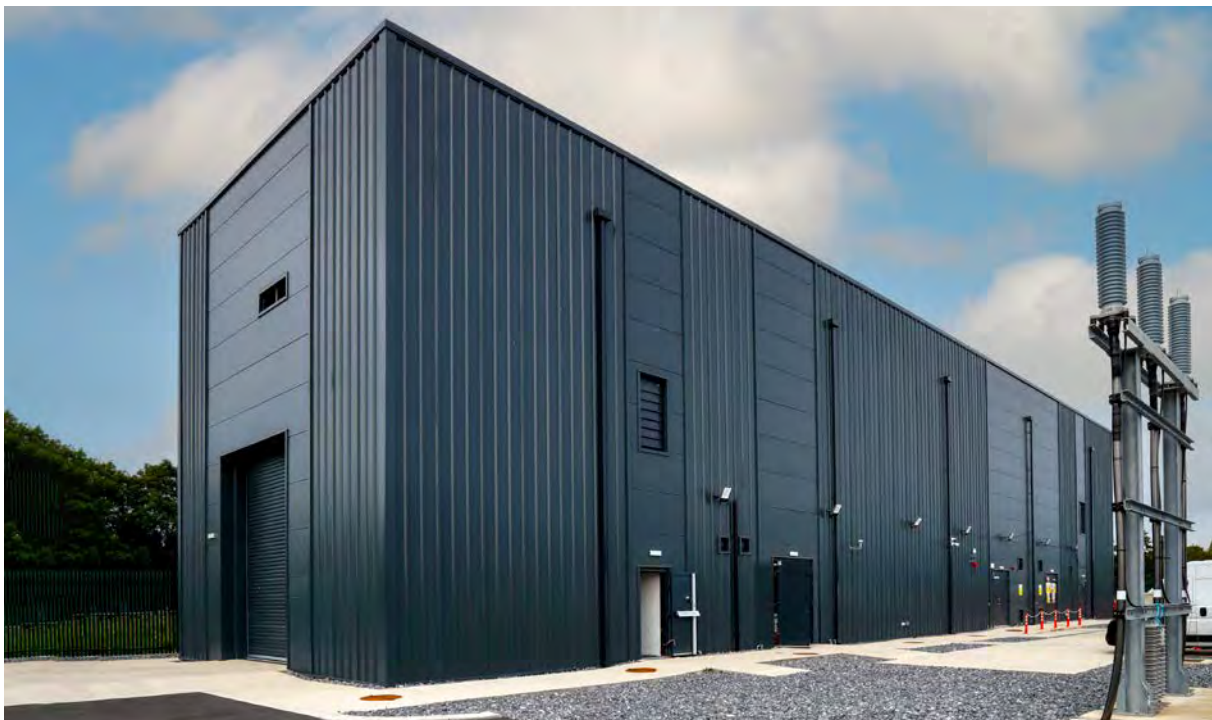
Figure 14: Typical GIS station
