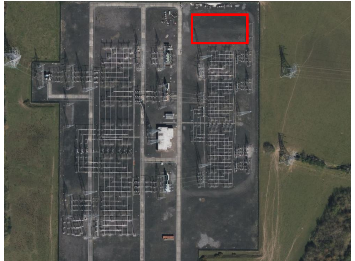
Woodland 400 kV Station
