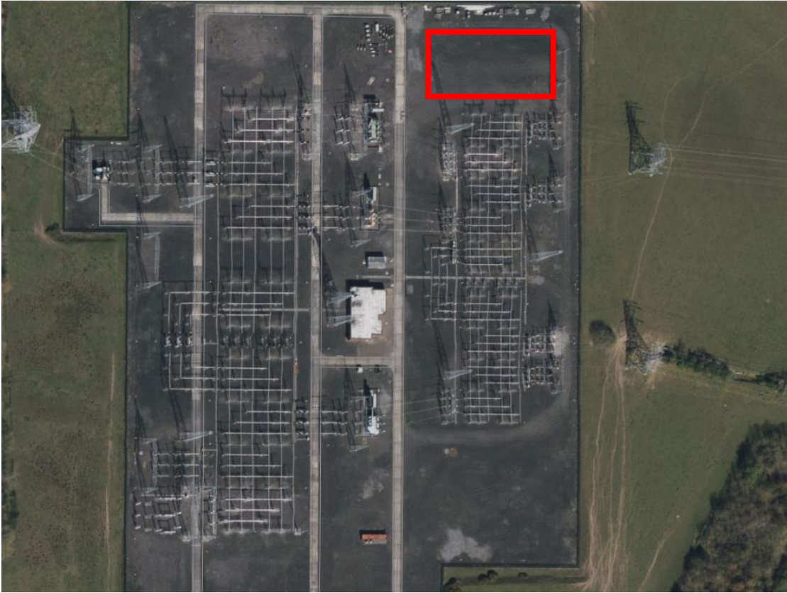
Woodland 400 kV Station
