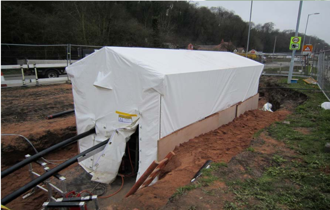
Figure 3.6 – Cable Jointing Tent
