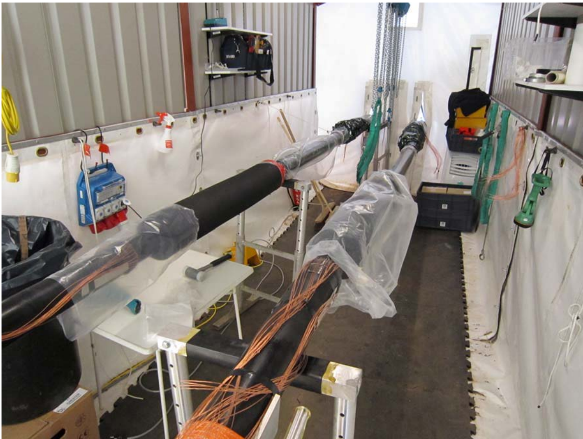
Figure 3.7 – Cable Jointing Tent
