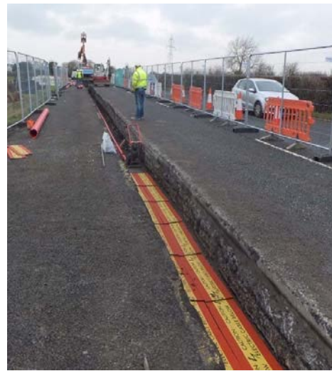
Figure 3.3 Cable Trench
