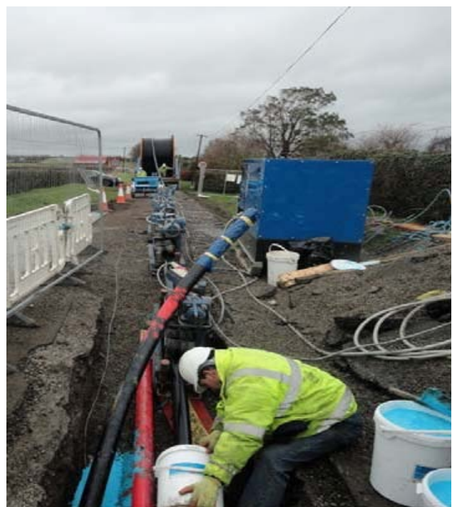
Figure 3.9 Cable Installation
