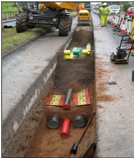
Figure 3.2 Cable Duct Installation
