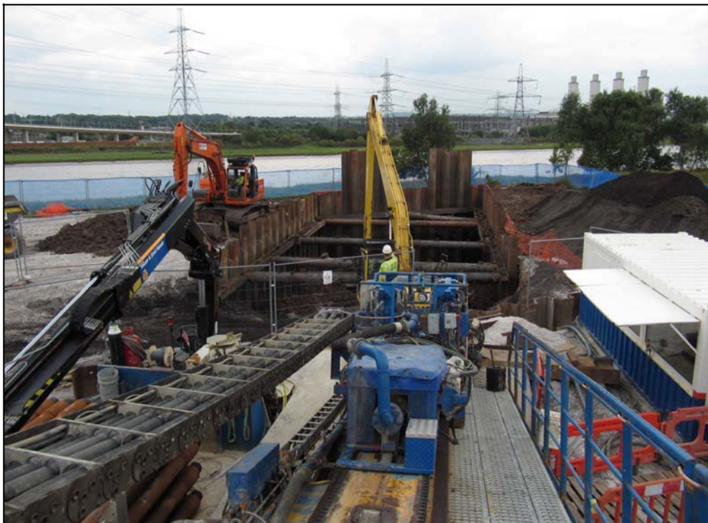
Figure 3.11 Example of Horizontal Directional Drilling rig (HDD)
